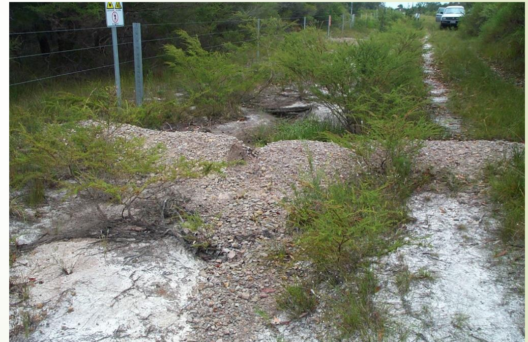
Poor construction, failed due to lack of volume and storage capacity
