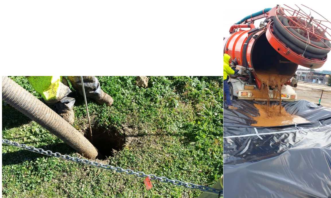
Figure 14. (Left) Non-destructive drilling (back-of-hole) and hydrovac (front-of-hole). (Right) Drillers mud being emptied from a hydrovac truck
