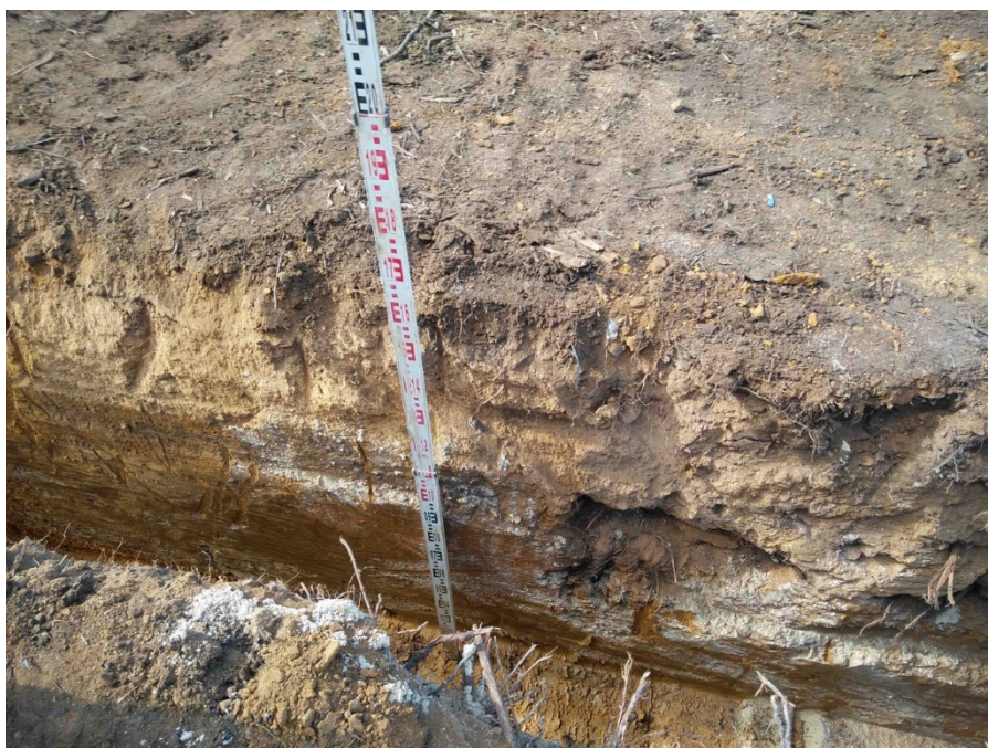
Figure 3. This trench had residual backfill sand material, common along the corridor where existing services are within vicinity
