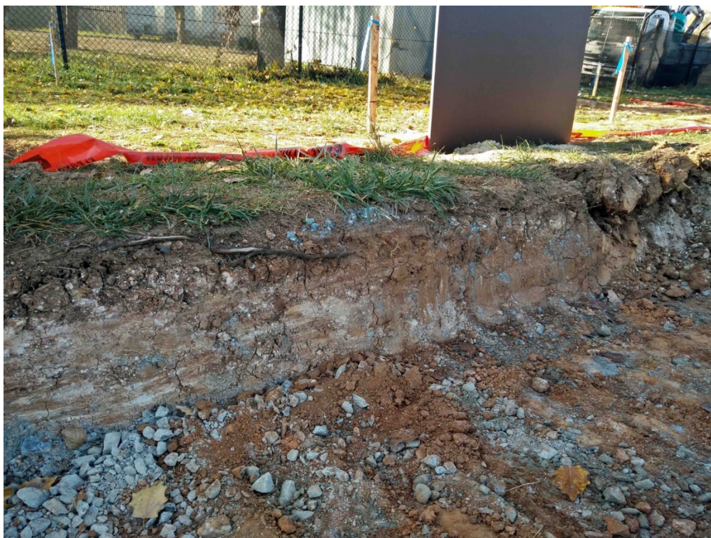
Figure 4. This was a road verge with fill material, hardly any suitable site soil resource for reuse
