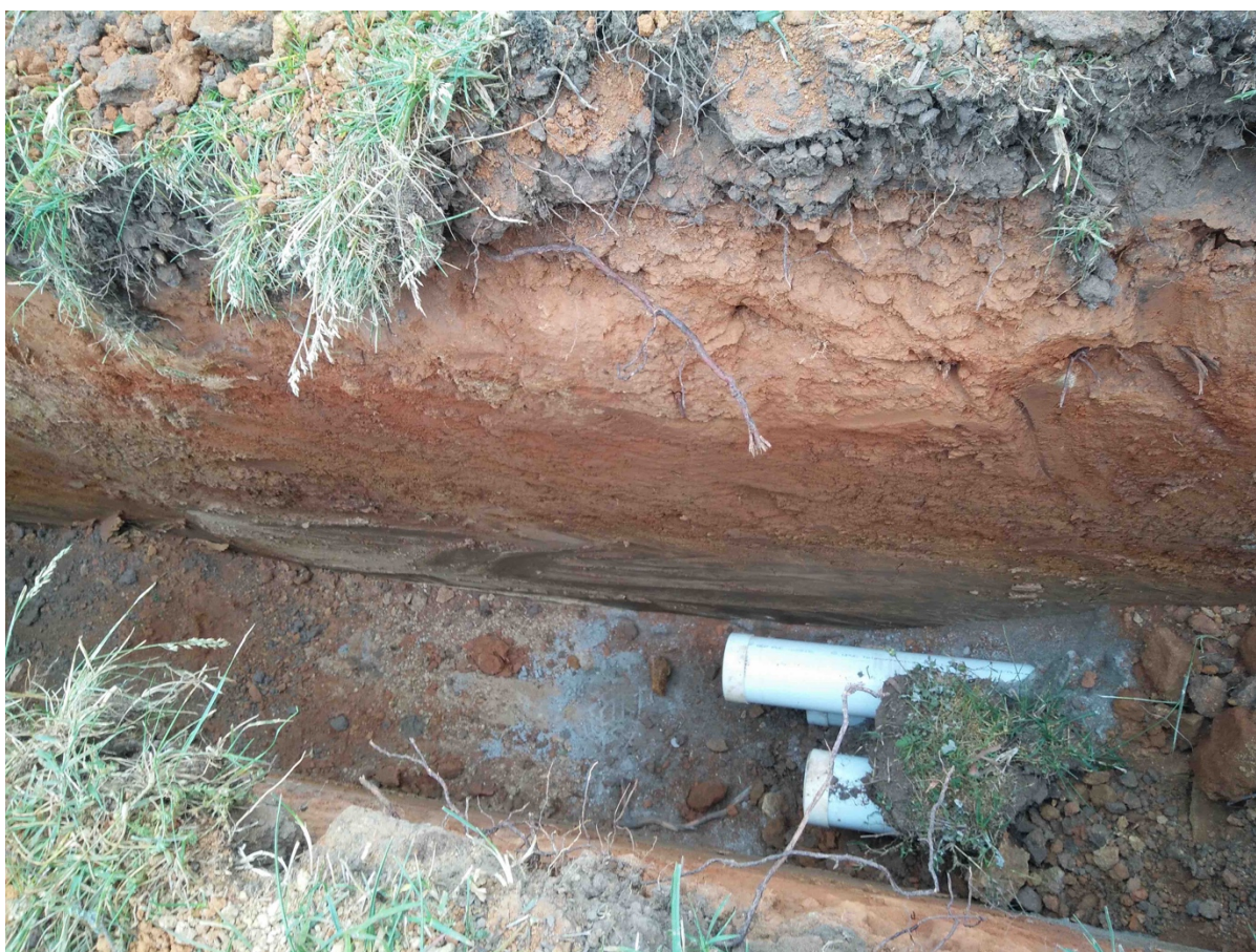
Figure 10. Trench with services and limited topsoil
