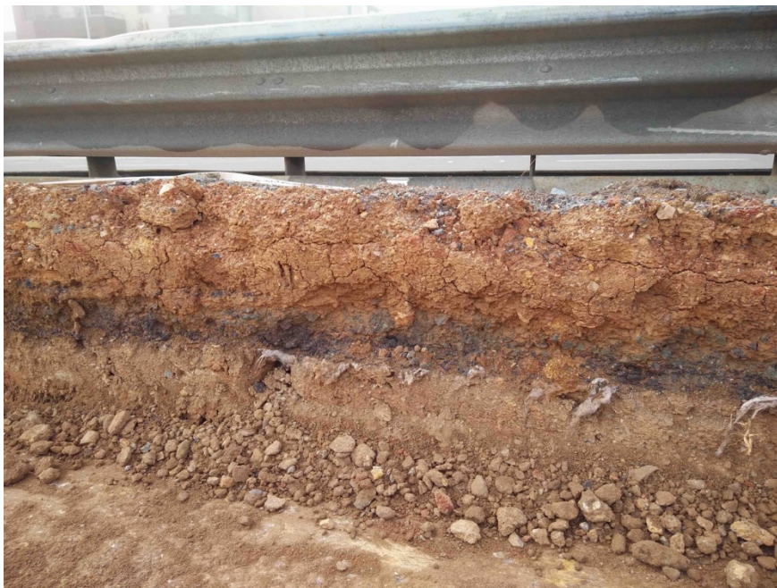
Figure 8. Imported fill with no topsoil under a slab in a part of the project area thereby limiting the soil resource available for reuse. A large portion of the project area where there was bulk earthworks was similar to this, hence limited available soil resource
