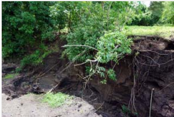
Erosion impact after January 2015 flooding in Ntcheu, Malawi. Photo: J. Braslow/CIAT
