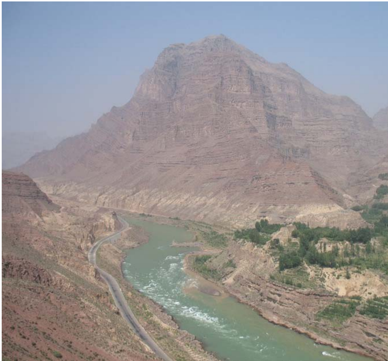
Jishi Gorge upstream the landslide dam. The grey silt deposits dozens of metres above the water level are lacustrine sediments.
