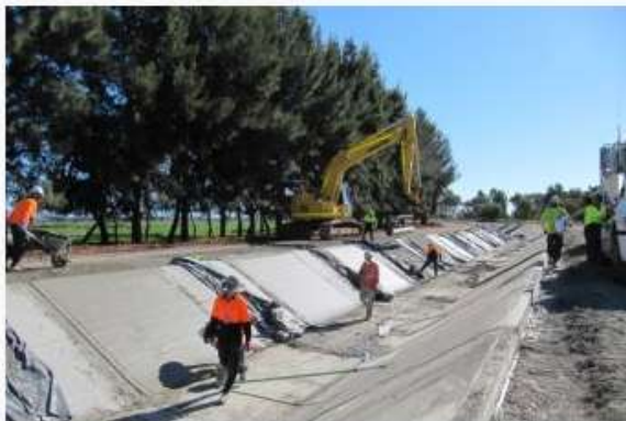
PHOTO: Channel upgrades have been part of Murrumbidgee Irrigation's $50m Lake Wyangan project. (Laurissa Smith)
