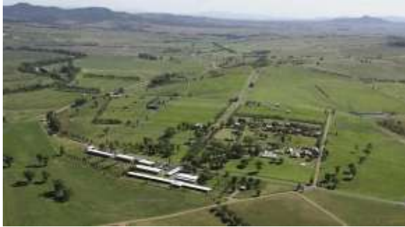
Saved from the coal mine expansion at South Drayton. Photo: Peter Stoop
