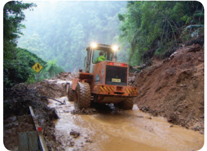
Mass movement of deeply weathered soils from road cutting: NSW North Coast.
