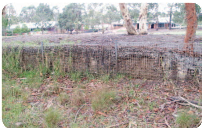
Erosion and deposition in an urban catchment: School playground, Rathmines, NSW.
